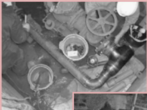
A newly installed 4" service line (above), and a new 16" butterfly valve (right).
