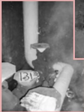
Recently repaired insulation for a 4" service line (above). A steam leak in a manhole before it was repaired (right).
